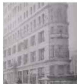
Panorama of Flatiron Building
